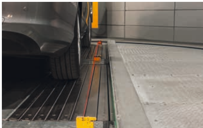
Lateral sensors are used in the transfer areas. Photo: Luis Sánchez Núñez de Cáceres
