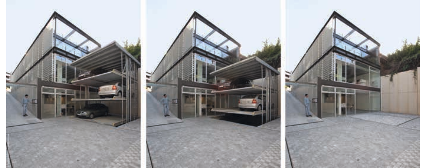
The automatic parking system is invisibly recessed into the ground. The horizontal, subterranean platforms only become visible when raised to provide access to the vehicles. The cover plate can be individually adapted to the local surroundings.
